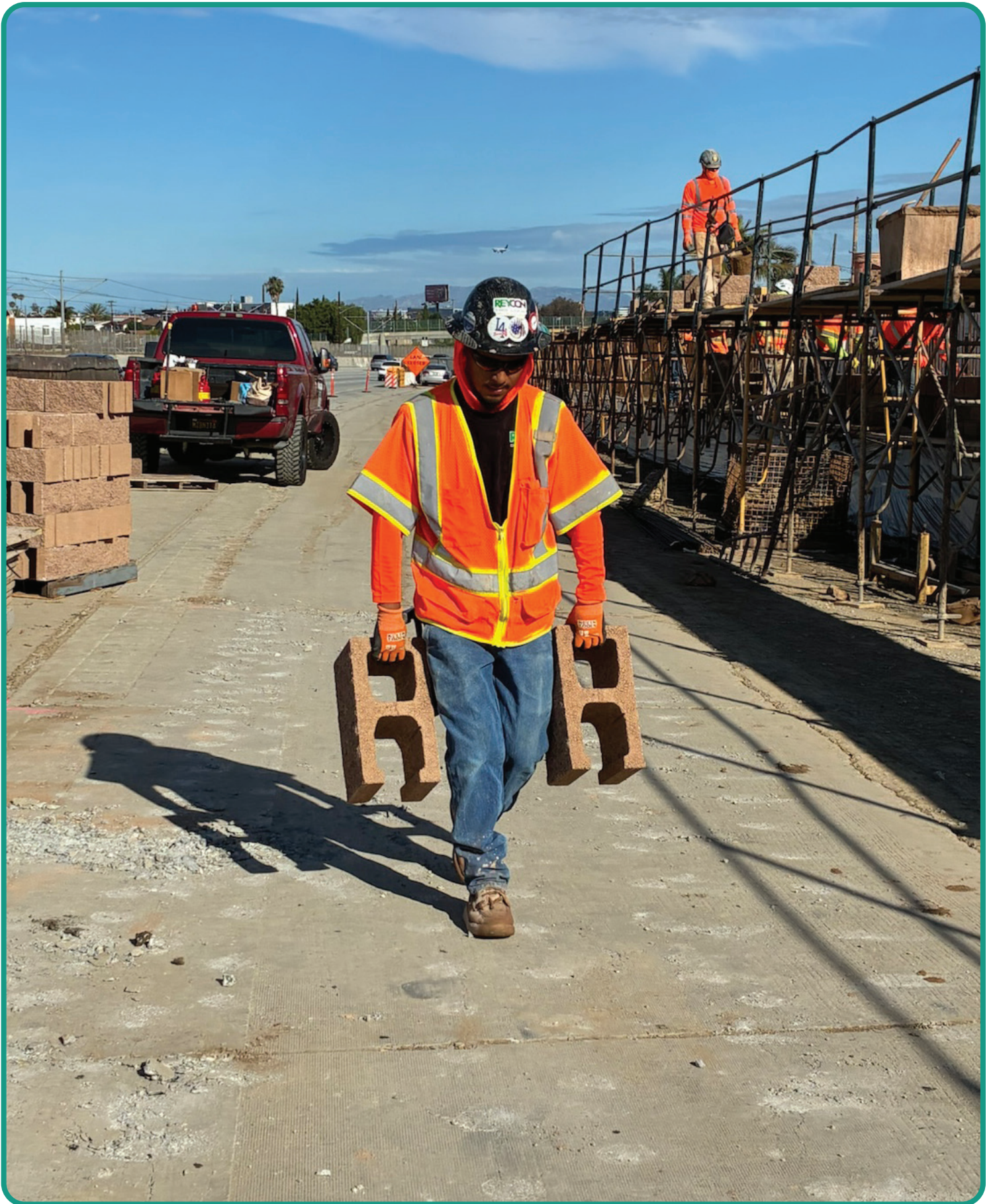
Block Wall Install
