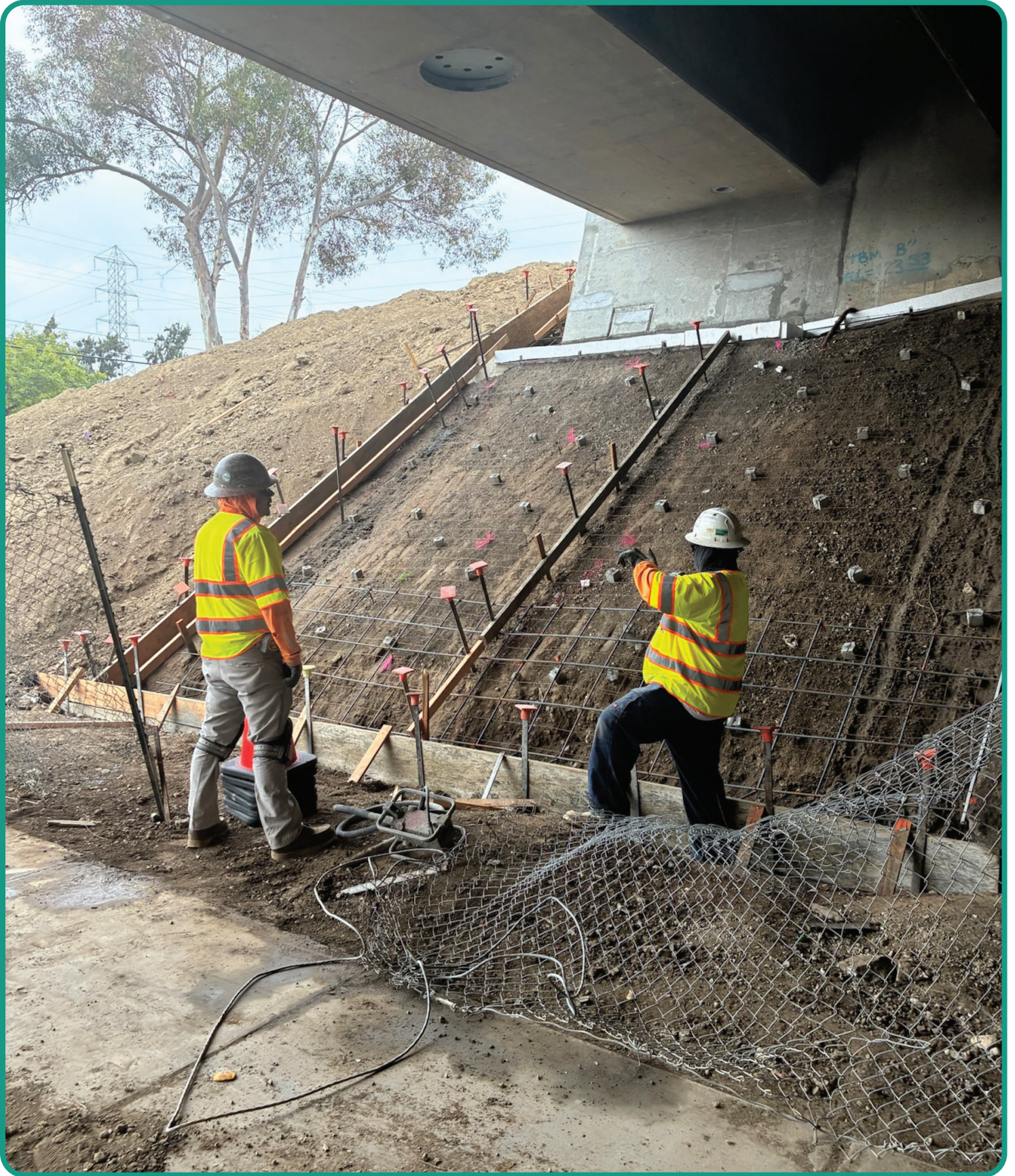
Slope under bridge
